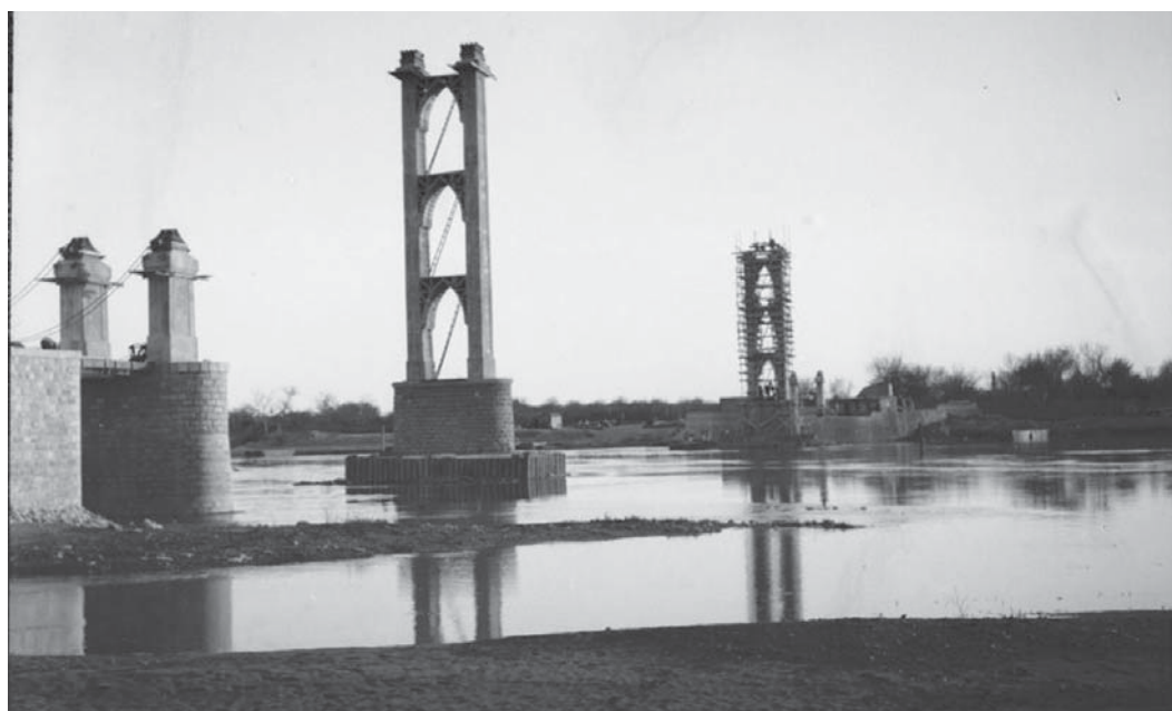
Fig. 6. The cable-stayed suspension bridge in Deir ez-Zor under construction, April 1928 (photo from the archives of the architect-archaeologist Maurice Pillet)
