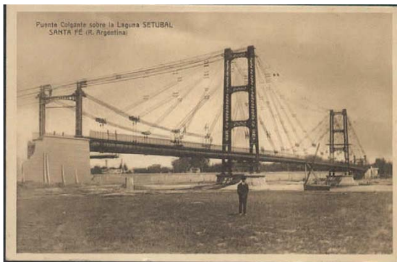
Fig. 12. “Puente Colgante de Santa Fe” bridge in Santa Fe, Argentina, with an improved radial cable-stayed truss of the Gisklard system (a circa 30s), (photo from the archives of Arnodin – Leinekugel Le Cocq)
