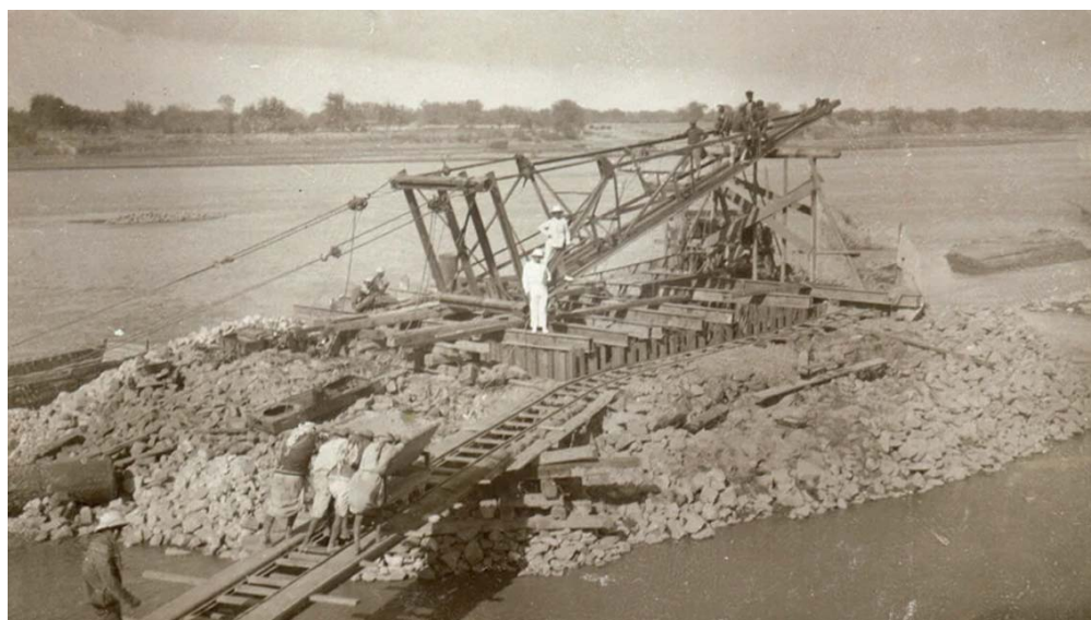
Fig. 4. The beginning of the construction of the cable-stayed suspension bridge in Deir ez-Zor, 1925. Installing a crane to erect a bridge pier (photo from the archives of Arnodin – Leinekugel Le Cocq)
