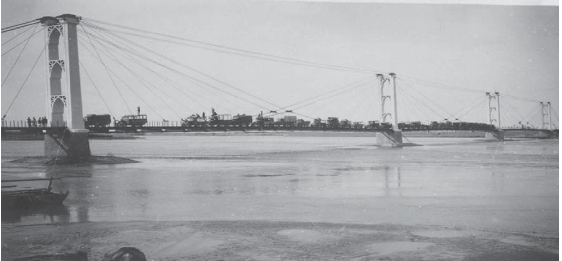
Fig. 7. Inauguration of the cable-stayed suspension bridge in Deir ez-Zor and testing the load bearing capacity of the bridge deck in 1931 (photo from the archives of Arnodin – Leinekugel Le Cocq)
