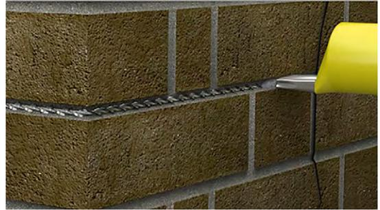
**Fig. 14.** Reinforcement of corner walls in the presence of cracks
